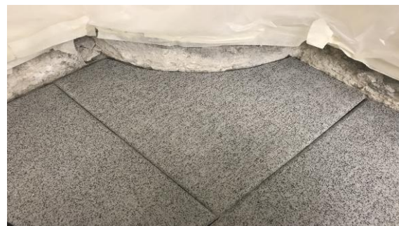
tiles can also be cut around curves
