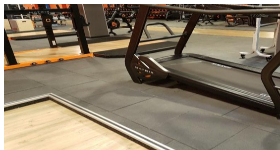
Perimeter step made by using a metal bar
