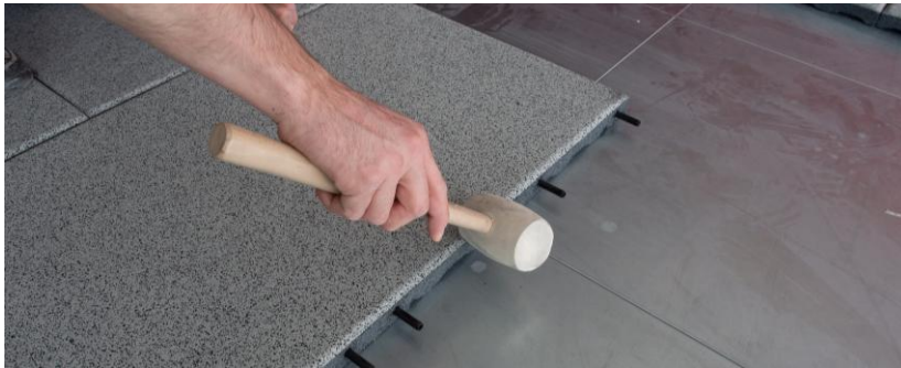
Closing the gaps with a hammer
