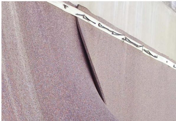
Mat secured to the wall using screw-fastened strips
